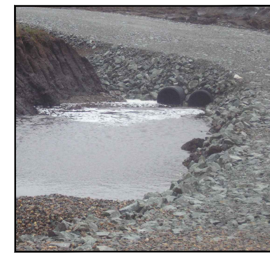
TYPICAL UNDER TRACK DRAINAGE
