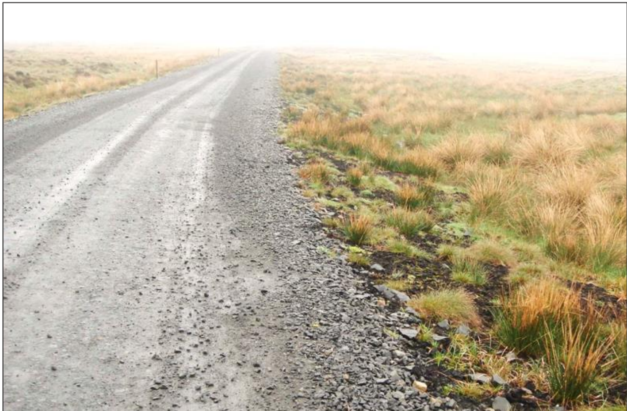
Figure 4.1: Example peat turf management with subsequent re-establishment of verge
